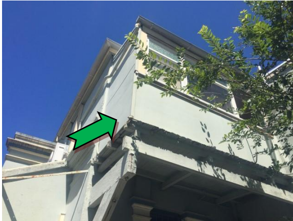
Photo 1. Exterior, level 1, external walls – assumed non asbestos-containing fibre cement sheeting.
