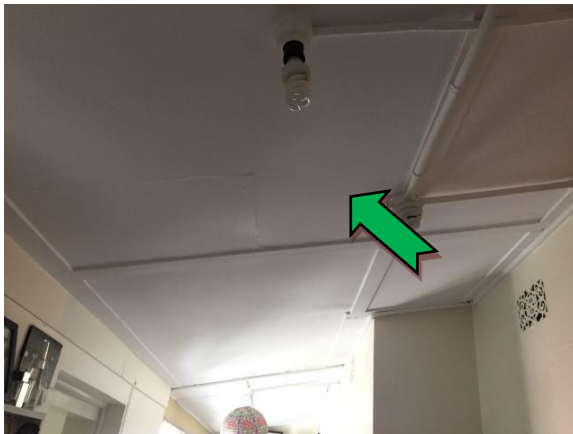
Photo 3. Level 1, western extension, ceiling lining – non asbestos-containing fibre cement sheeting.
